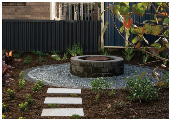
Blocks arranged in stretcher bond pattern
